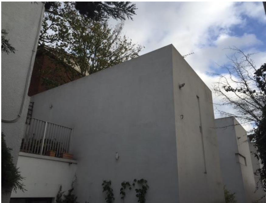
Image 6: View of existing flat roof of no. 4 from west of site
