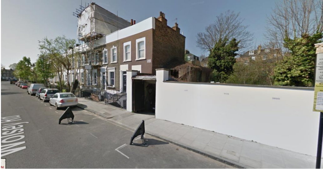
Image 3: View looking south on (Wolsey Road)
