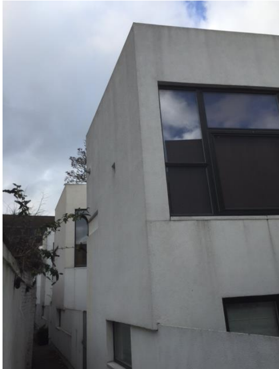
Image 7: View from access path towards site
