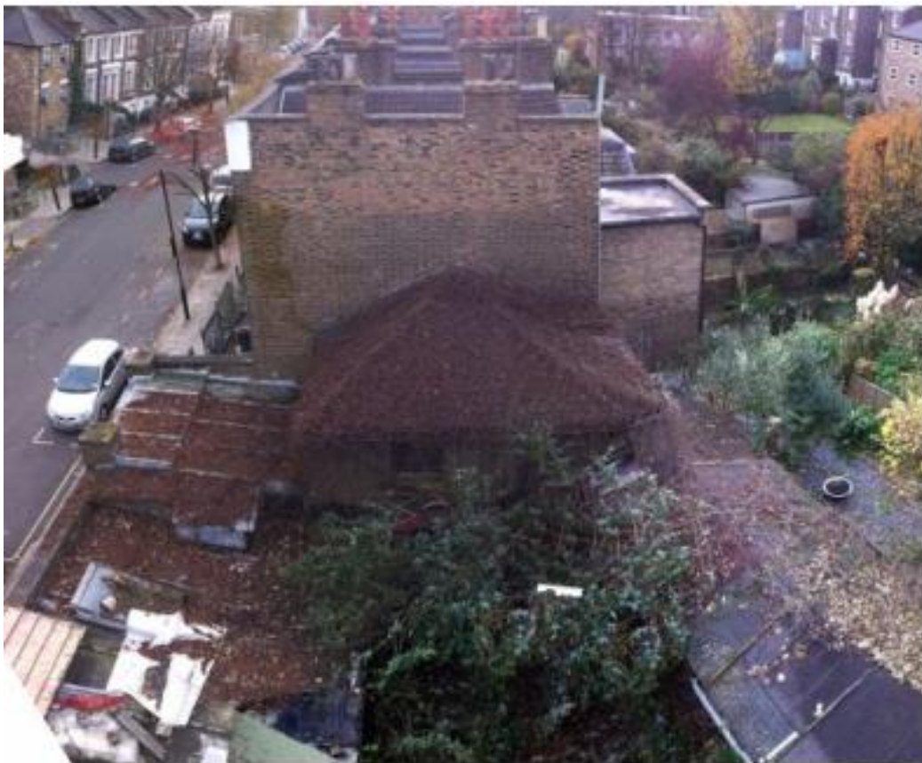
Image 4: View from the rear of 121 Mildmay Road.
